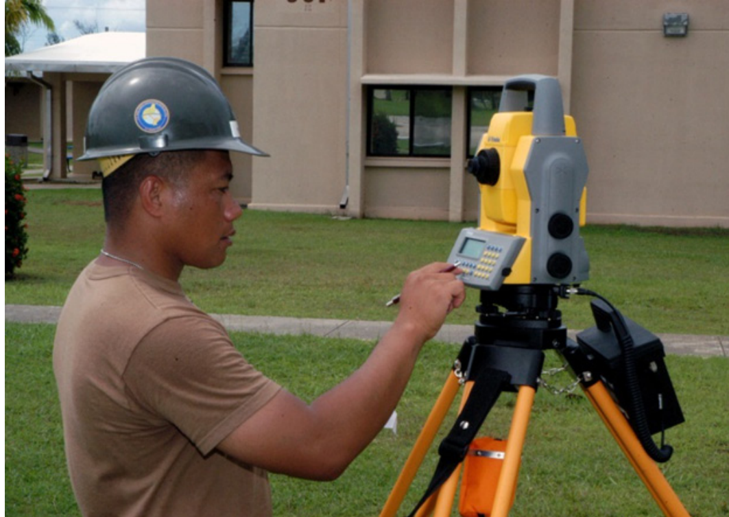
Figure 7.9. Surveying with a Total Station
